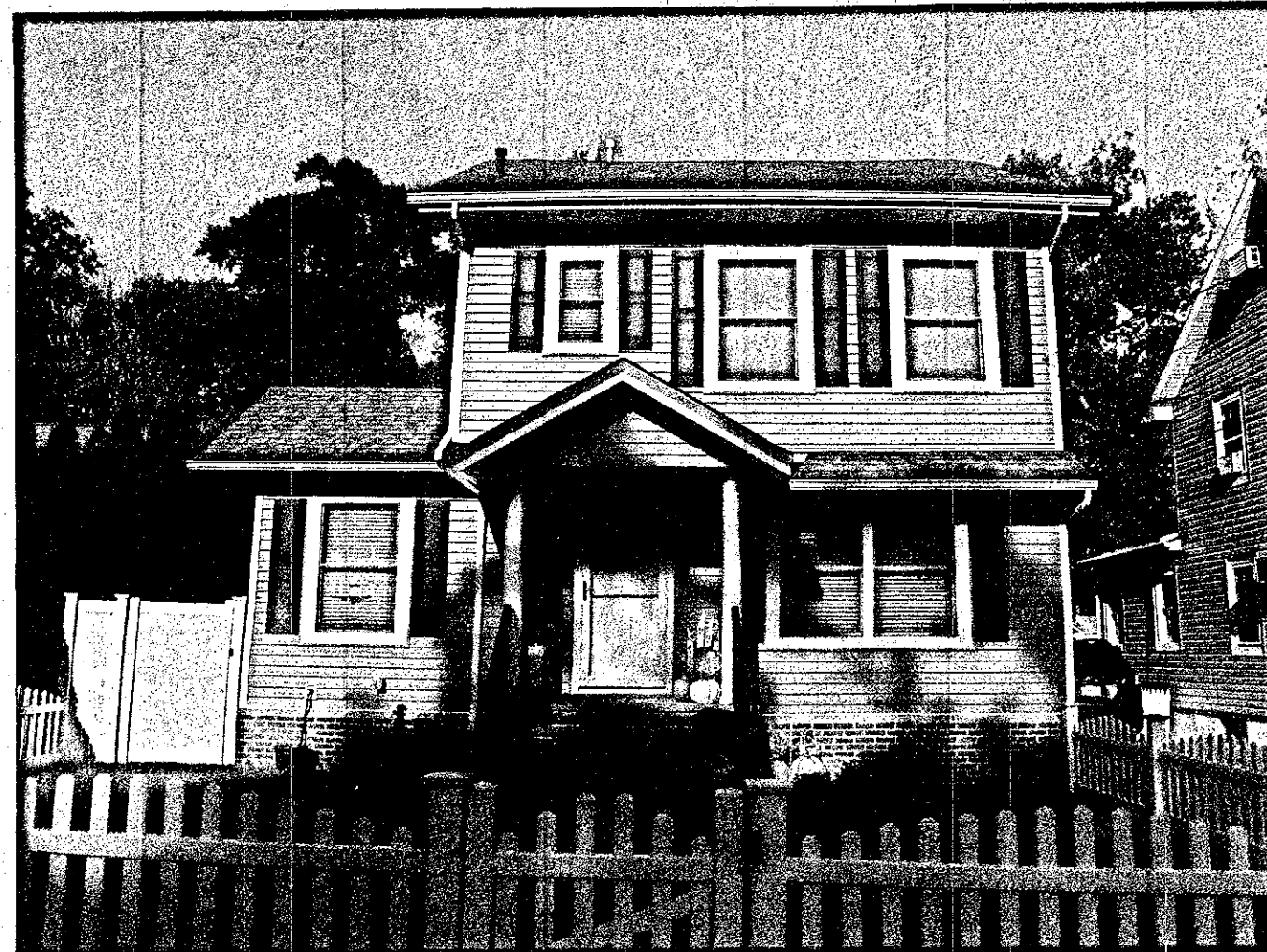
PH-1 - VIEW OF FRONT (EAST) ELEVATION - GROVE AVENUE
